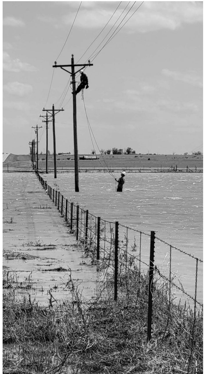
▲ Outage restoration in Baca County area after recent storm.
