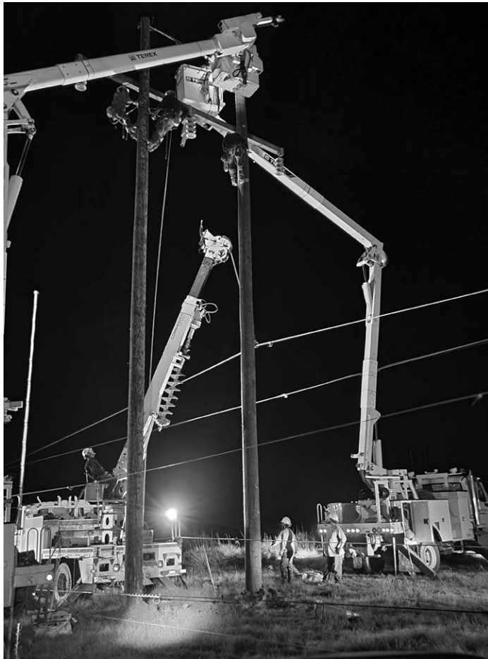
▲ Crews work through the night rebuilding a storm-damaged structure.
